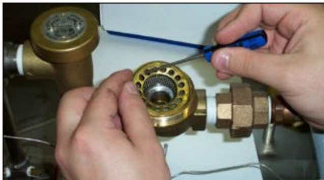
Removing the screen retainer
