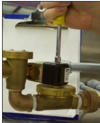
Removing the top screw
