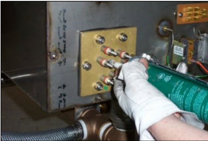
Applying silicone to the heater well
