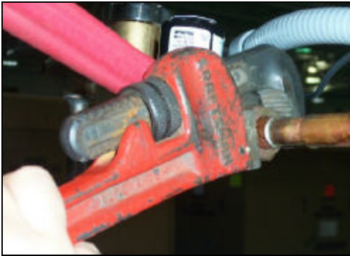
Loosening the union on the incoming plumbing
