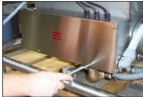
Removing the heater box cover
