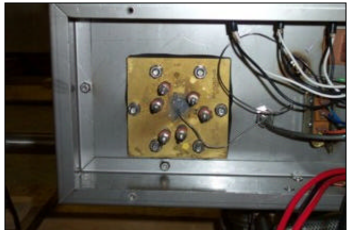
Heater without power lines attached.
