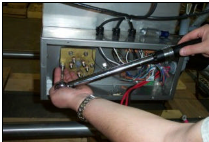
Applying the torque wrench to the nuts
