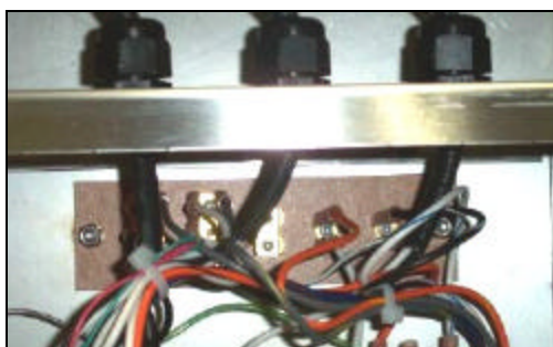
Terminal board inside the heater box
