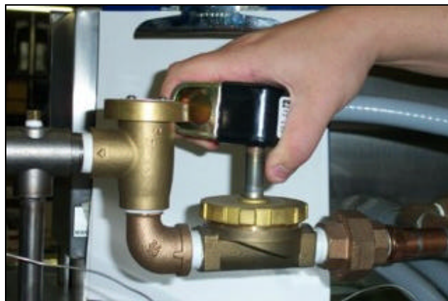
Removing the coil
